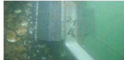
Installation of Al anode for offshore steel pile
