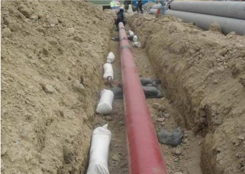
Installation of Mg anode for U/G piping
