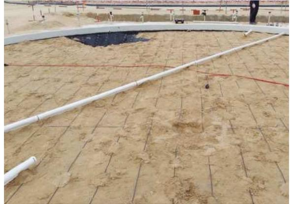
Installation of MMO-Ti ribbon anode for tank bottom
