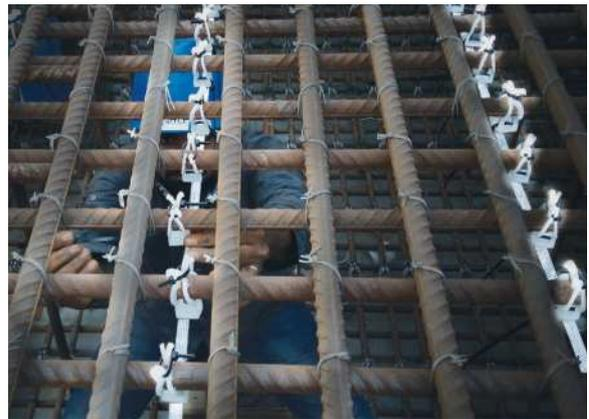
Installation of MMO-Ti ribbon mesh anode for concrete rebar
