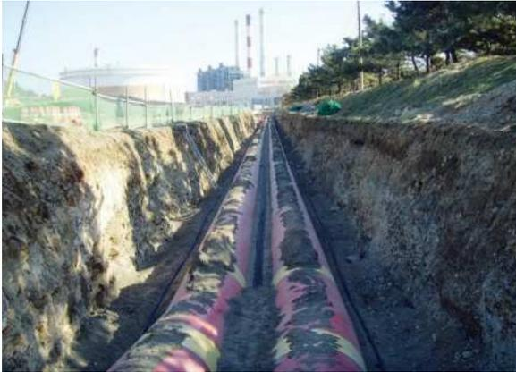
Installation of liner anode for U/G piping
