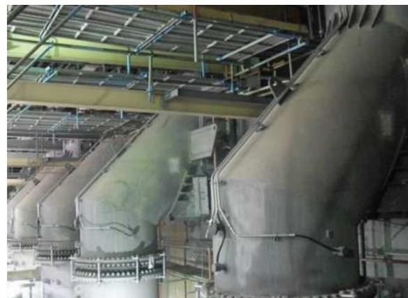
Installation of Pt-Ti anode and ref. electrode for condenser
