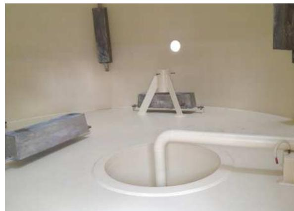
Installation of Al anode for tank internal
